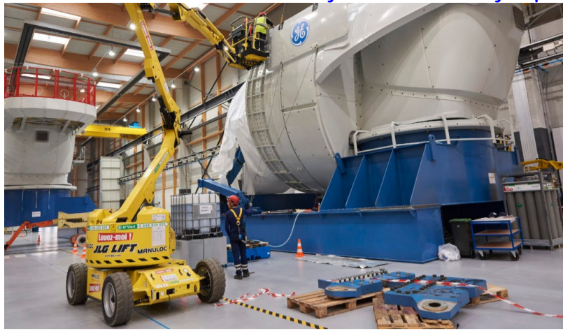
The nacelles during production in the Saint-Nazaire factory. Image credit: GE Renewable Energy
